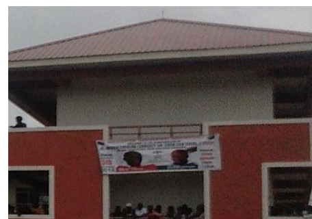
The State funded project covered with NDC Banner during the Commissioning
